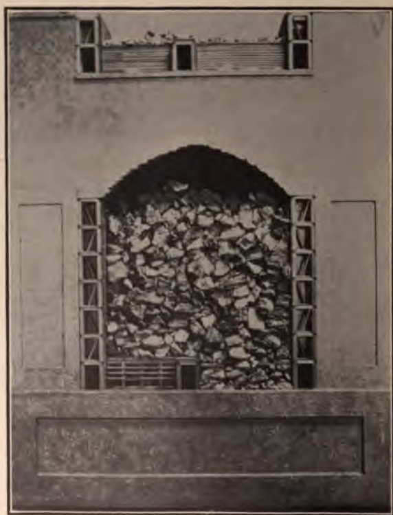
Fig. 37.—End View of Stope in Homestake Mine, Back-filling Method. From Model in Engineering Office of Company.
